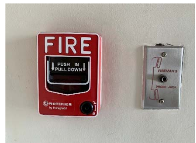
Fire Alarm Manual Station
